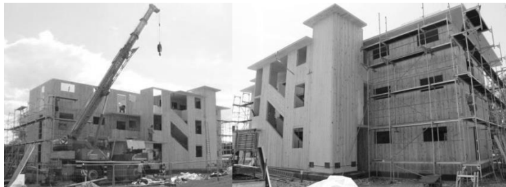
Figure 1. Site of investigated object during construction (Eder 2015).
