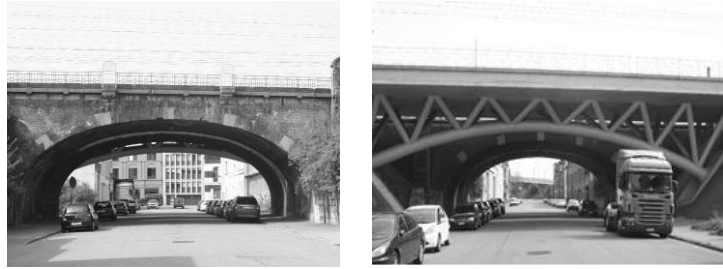
Figure 1. The existing MSB before refurbishment ( right ); the new MSB for the high-speed railway line ( left ).
