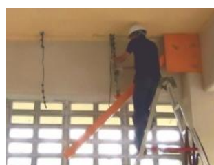
(e) Replace with the wire rope.
